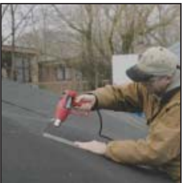
Weld Roofing Felt
