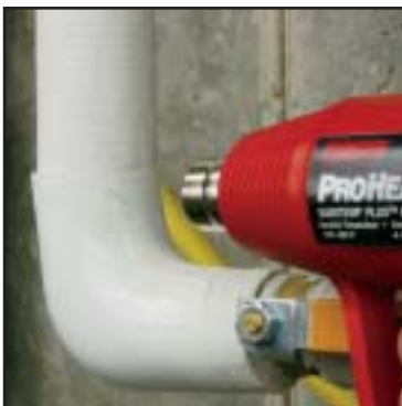
Dry/Seal Insulation
