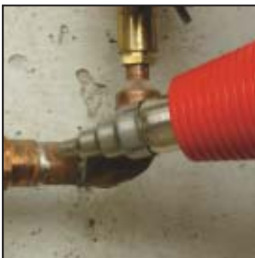
Solder Copper Pipe
