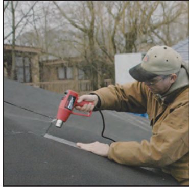
Weld Roofing Membrane
